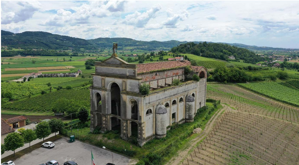
Fig. 1: Overview of the “Unfinished” church of Brendola.
